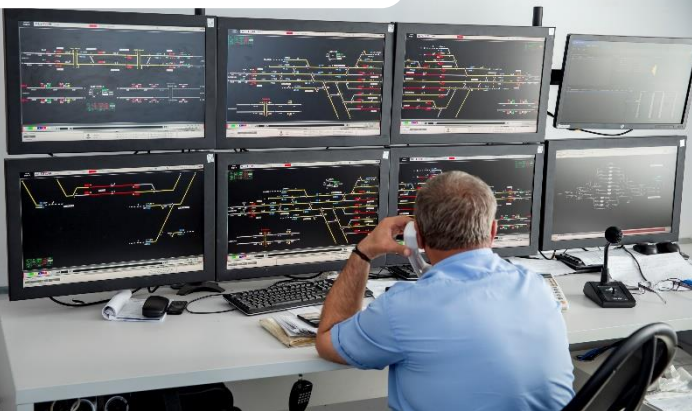
Digital traffic management centre in Arad
