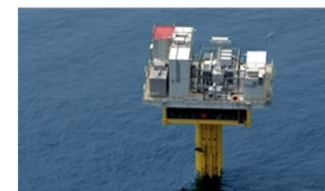
Offshore substation in Europe
