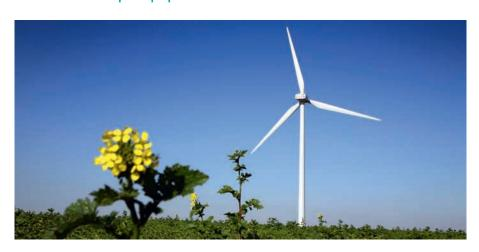
With a power output of 3 MW, the Eco100 is the most powerful onshore wind turbine on the market. At 140 metres high, the equivalent of a 50 storey building, and with a rotor diameter of 100 metres, in which could fit the wingspan of an Airbus A380, the Eco100 is a new asset for Alstom in the field of renewable energy.
