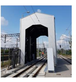
**24 November 2019** – Alstom's predictive maintenance solution for rolling stock, TrainScanner, has entered in service in Warsaw's Pendolino Service Centre, where it will be used to maintain the fleet of 20 Avelia Pendolinos operated by PKP Intercity.
